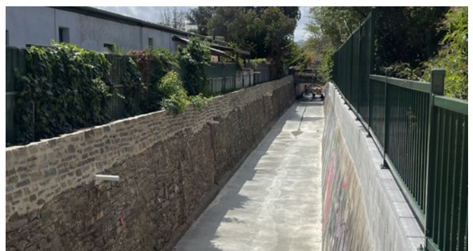
Leah St to Ethel St - Raised channel walls
