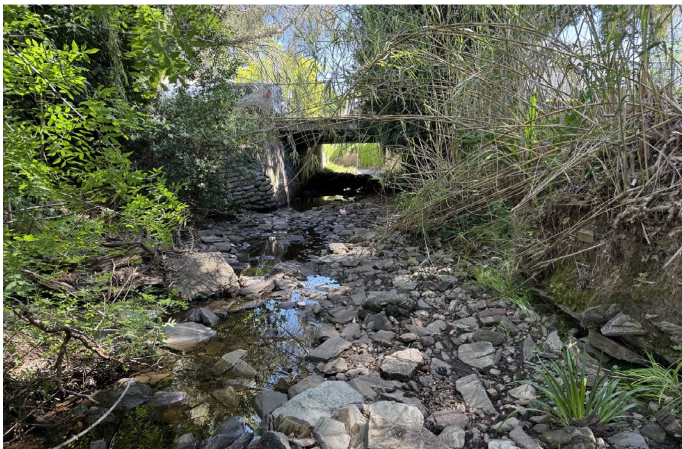
Orphanage Park - Existing Crossing
