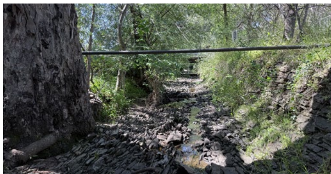
Orphanage Park - Existing Channel
